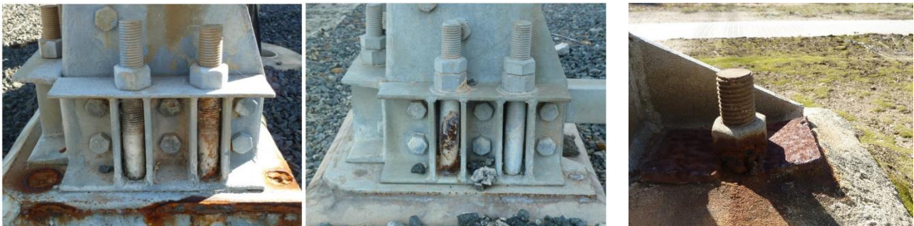
Figure 6 – View of typical corrosion of member connection bolts
