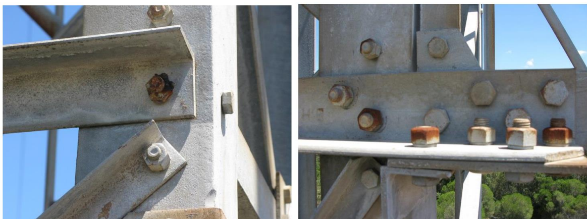
Figure 6 – View of typical corrosion of member connection bolts
