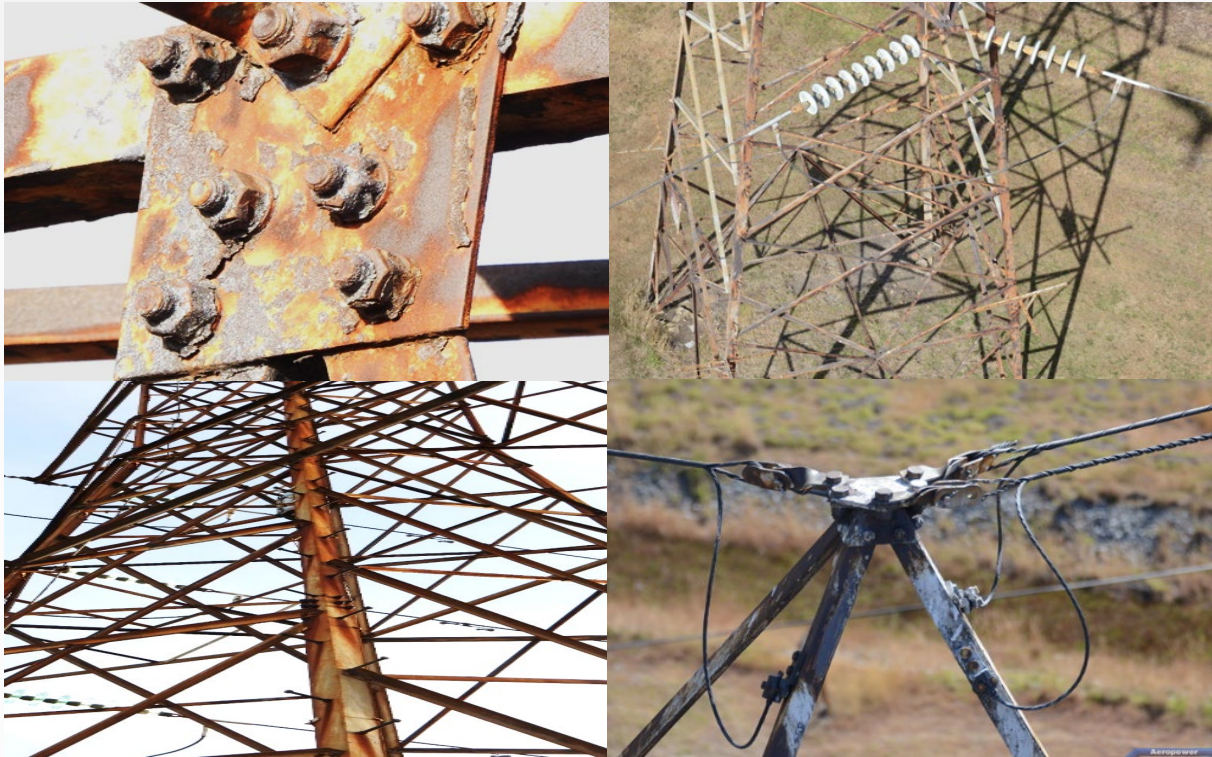
Figure 3: Typical tower condition
